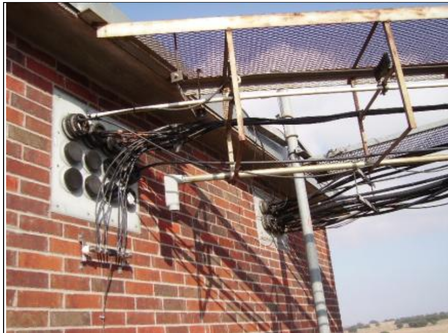
Mills County Coax, Ice Shield, & Grounding
