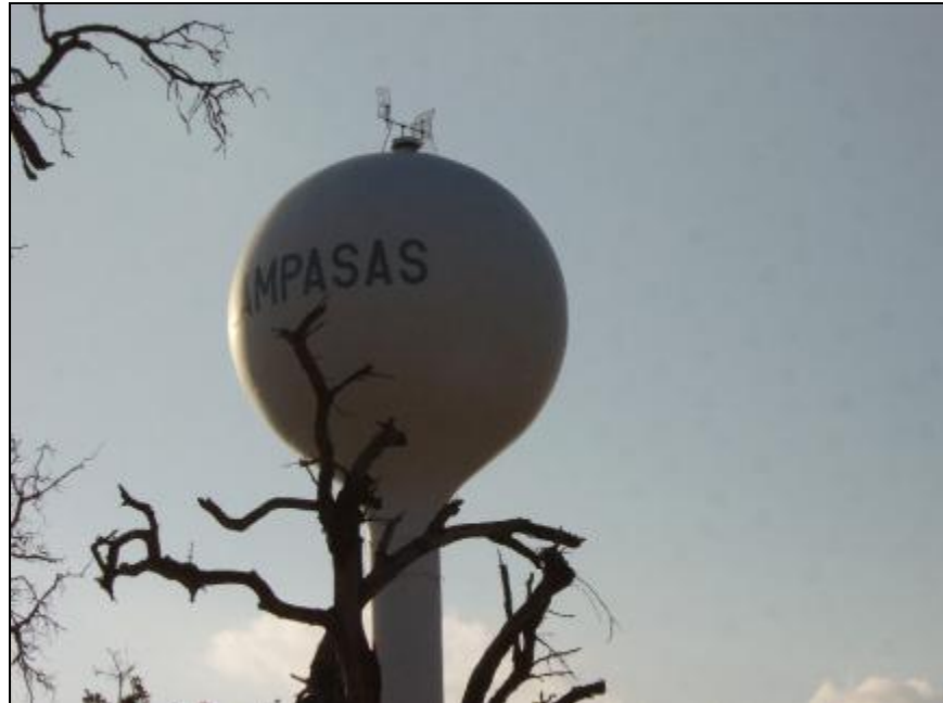
Lampasas Water Tower Microwave Link
