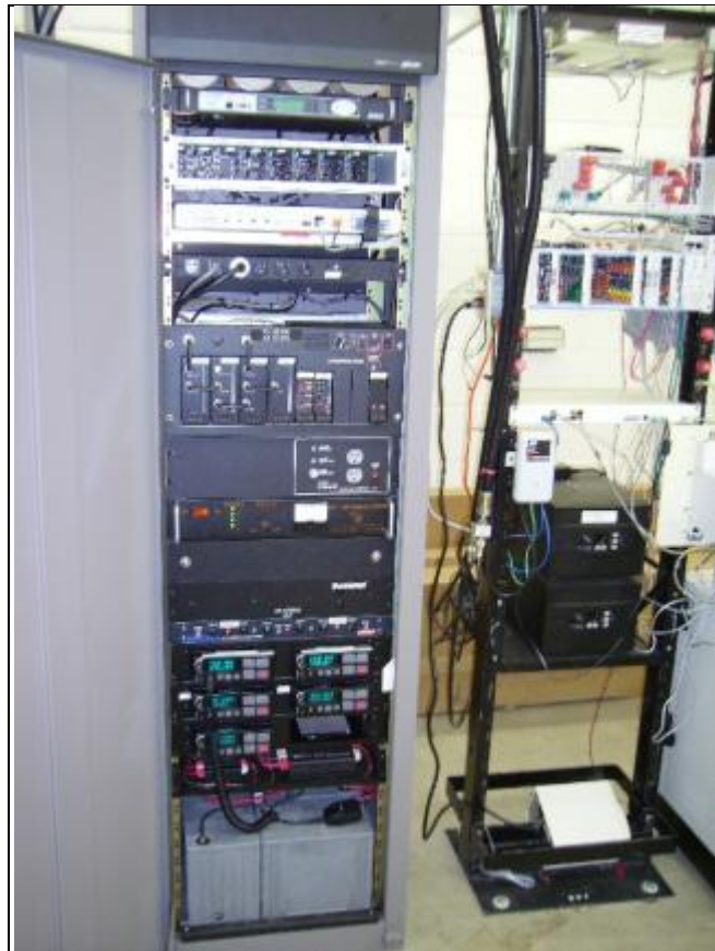
San Saba Microwave, Radio, Battery Equipment Rack
