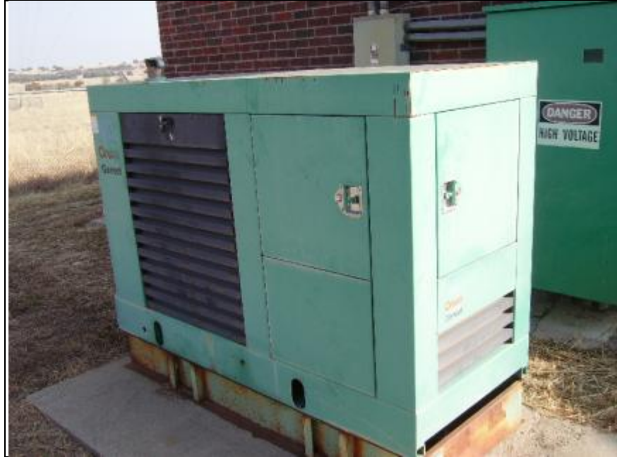
Mills County Backup Power Generator
