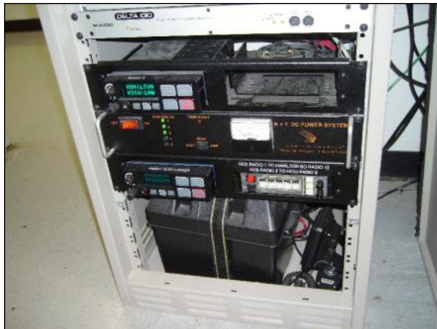
Hamilton County Radio with Power Supply & Battery
